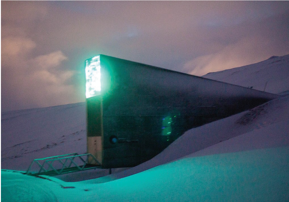
Figure 1.11. Svalbard Global Seed Vault. Source: https://commons.wikimedia.org/wiki/Category:Svalbard_Global_Seed_Vault#/media/File:Svalbard_Global_Seed_Vault_(16064027324).jpg
